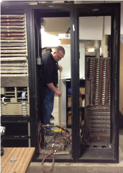
Harding Instruments Intercom System Panel – before and after the intercom system retrofit.
